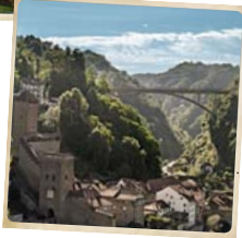
Galtertal bridge, Fribourg Region
